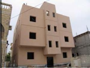
BPC has just completed the erection of panels on a 3 storey complete precast building. BPC has designed, produced, supplied and erected load bearing pigmented precast panels, hollowcore slabs and stair cases.
