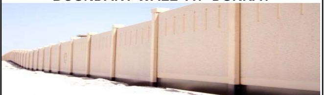
This is a 3.6 km long boundary wall coming up in Durrat. Design and Production, of 120mm thick pigmented solid panels for the
