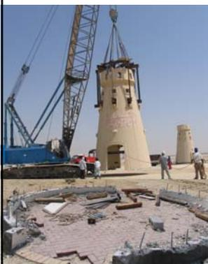
A big advantage of precast panels is recently experienced in the form of its modularity. A precast structure was erected about 4 years ago in Endurance Village. The owners wanted the structure to be moved 100 meters away from its place. BPC disconnected the structure from its base, moved to its new place and re-erected at
