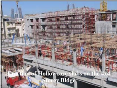
Erection of Hollowcore slabs on the 4x4 Storey Bldge
